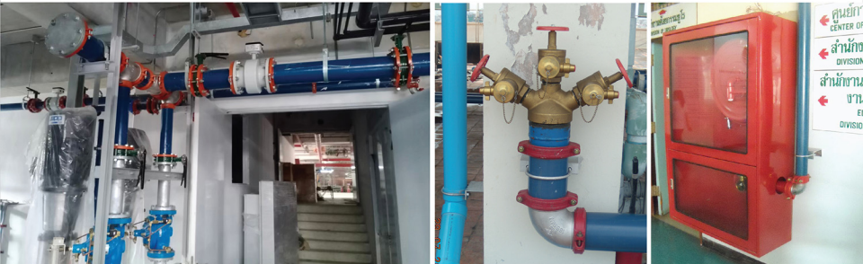
Figure of PRV installation with SYLER pipe
