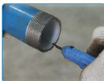
Scraping or trimming the pipe end
