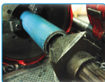
Trimming the pipe end with tapping machine
